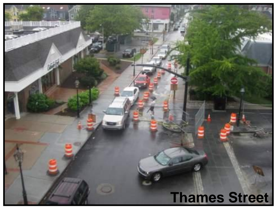
Typical Setup Size With a Short Work Zone with Barrels/Cones Short Duration Setups
