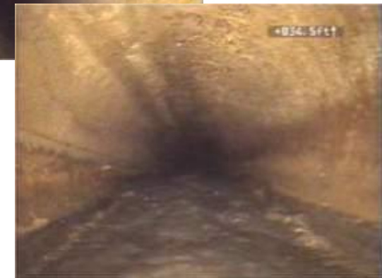
Spalling concrete pipe
