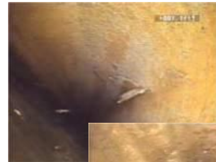
Spalling concrete pipe
